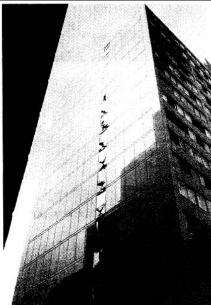
Classic shear failure of the coupling beams between linked shear walls at the south end of the building. (Hew et al., 1994)
