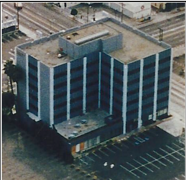
Aerial view of the Northeast corner of the building. (Comartin, 1999)
