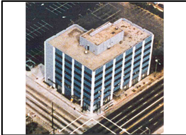
Aerial view of the Barrington Medical Building. (Comartin, 1999)
