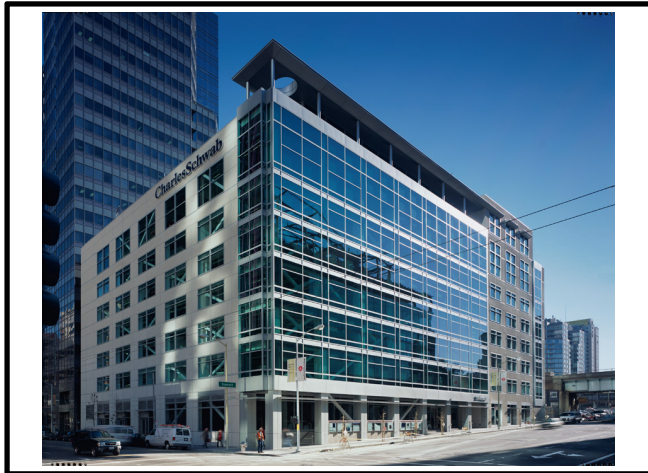
Elevation view of 215 Fremont Street, post retrofit. (Louie International, 2011)
