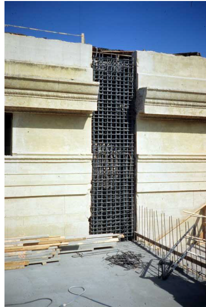
Installation of new reinforced concrete column in the museum lobby. (Poland, 2006)
