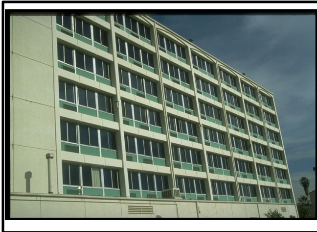
North elevation of the Van Nuys Holiday Inn prior to damage from the Northridge Earthquake (Clark, 1994).
